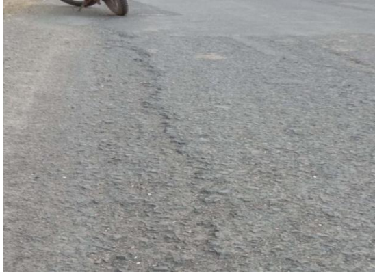
Fig.2 Transverse cracking
